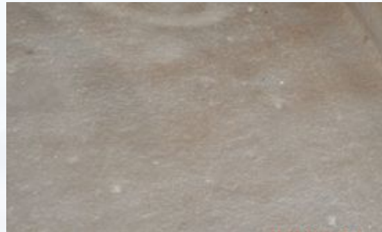
Full Abrasive grit blasting
