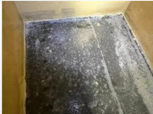
UHP water blasting
