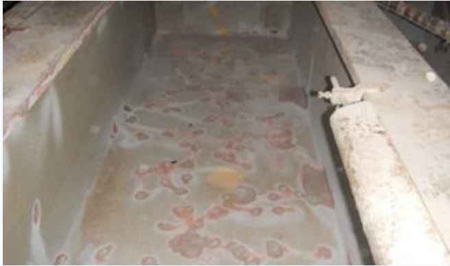
Abrasive grit blasting – pre-blast
