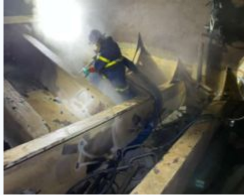
UHP water blasting
